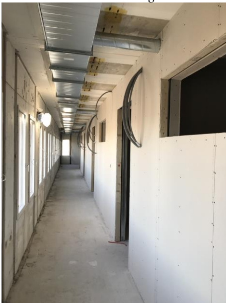
Ventilations installationer
